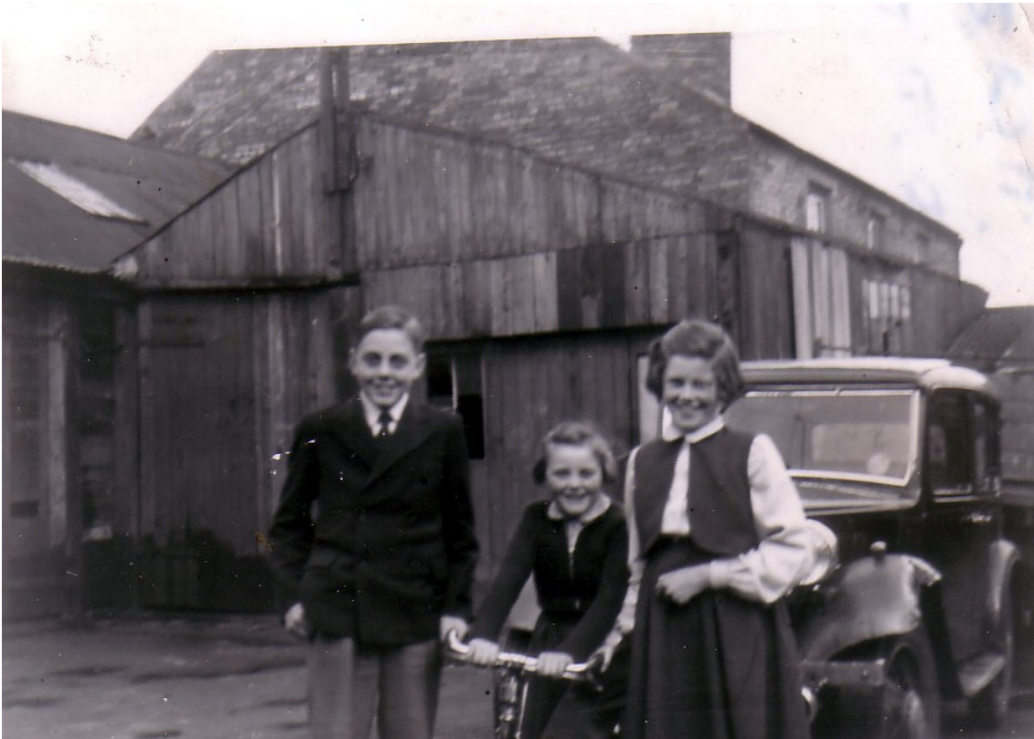
BRIDGE END GARAGE REPAIR WORKSHOPS AT THE REAR OF BRIDGE STREET, NEAR GARDEN PLACE
