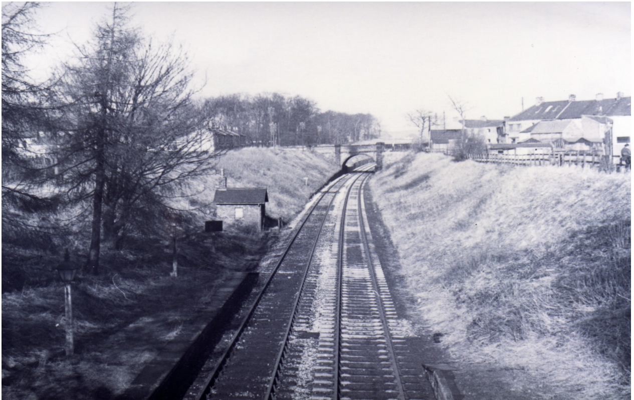
STEEP GRADIENT TO CROOK PASSED THROUGH THIS DEEP CUTTING All now infilled and reclaimed by DCC The fine stone bridge carried Bridge Street traffic over the tracks. Railway Street on the left
