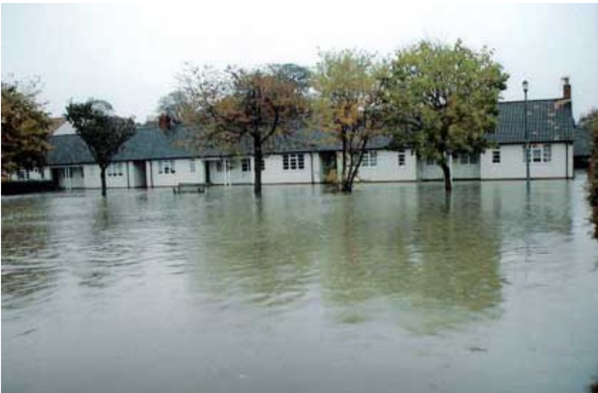
HOWDEN BECK FLOODS 30th OCTOBER 2000 LED INDIRECTLY TO THE DEMOLITION OF THESE AGED PEOPLE'S BUNGALOWS IN HARGILL HAVEN
