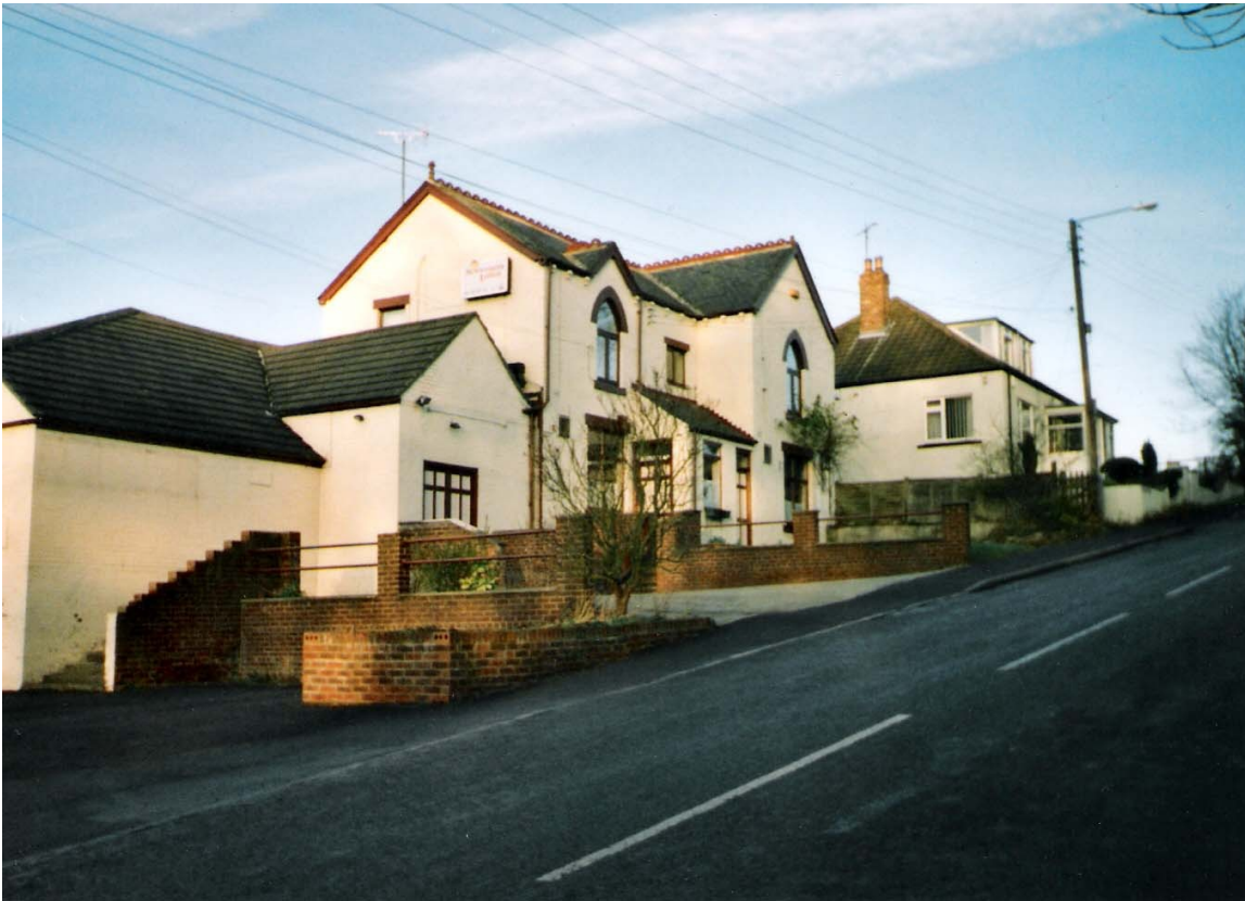
SUNNYDENE LODGE, FORMER WORKMEN'S CLUB, PRIOR TO DEMOLITION AND NEW HOUSING DEVELOPMENT c.2005
