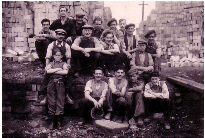
BRICKYARD WORKMEN c.1950s
