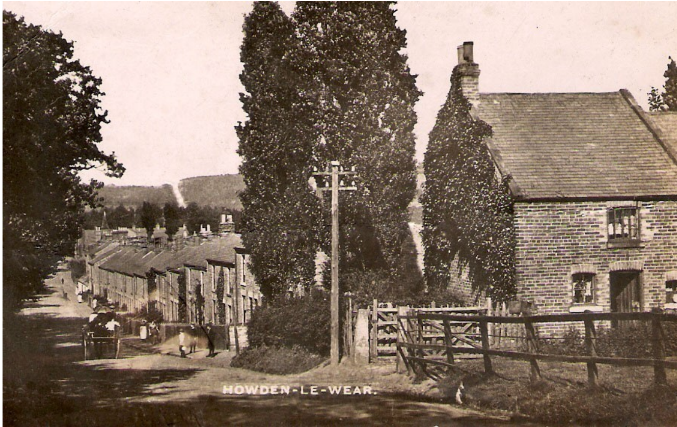
HARGILL ROAD WITH THE ORIGINAL HARGILL FARMHOUSE ON THE RIGHT
