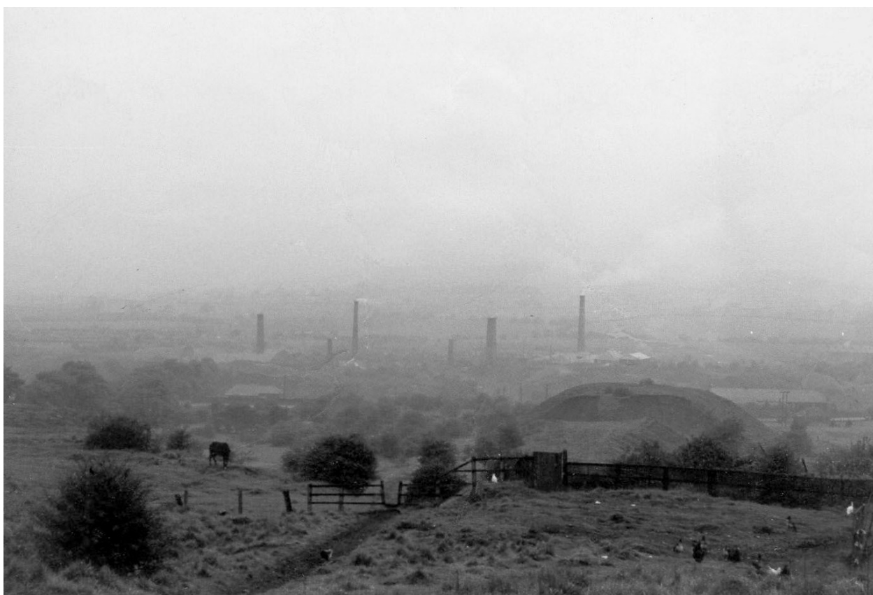
NORTH BITCHBURN COLLIERY COMPLEX LOOKING DOWN THE 'NAXIE' FROM NORTH BEECHBURN
