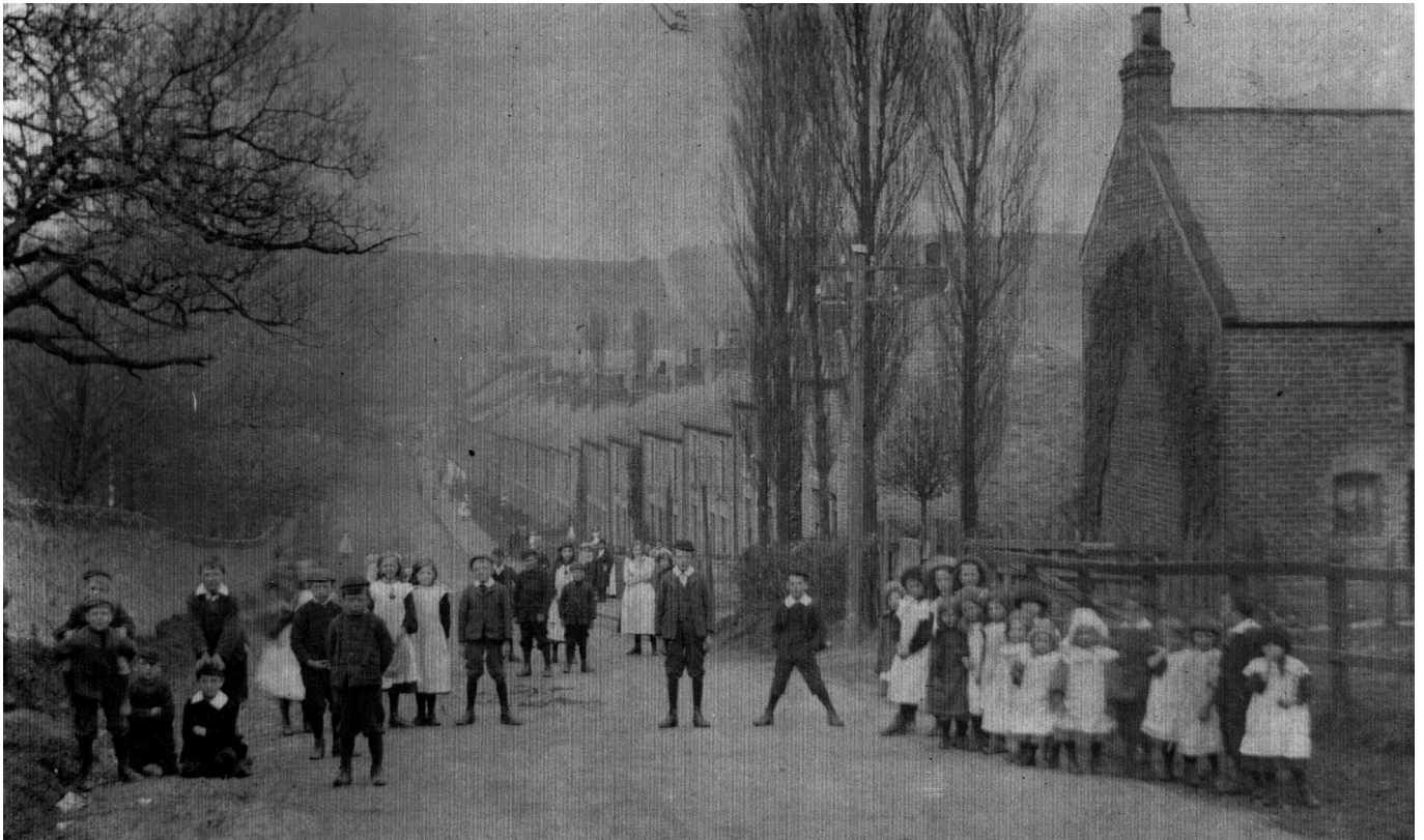
HARGILL ROAD EARLY 1900s
